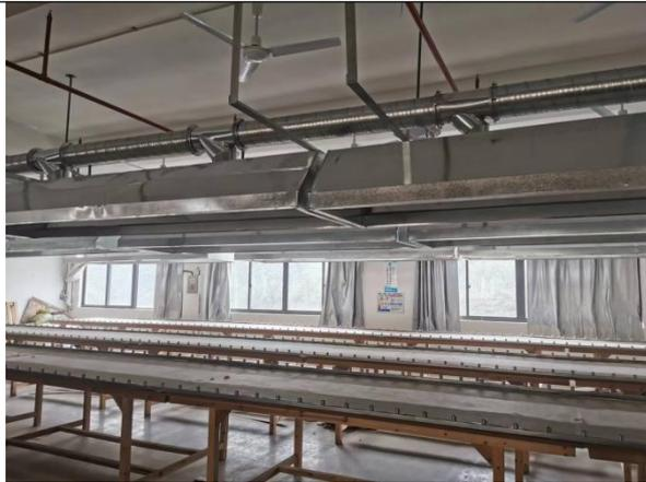
丝印废气集气罩
